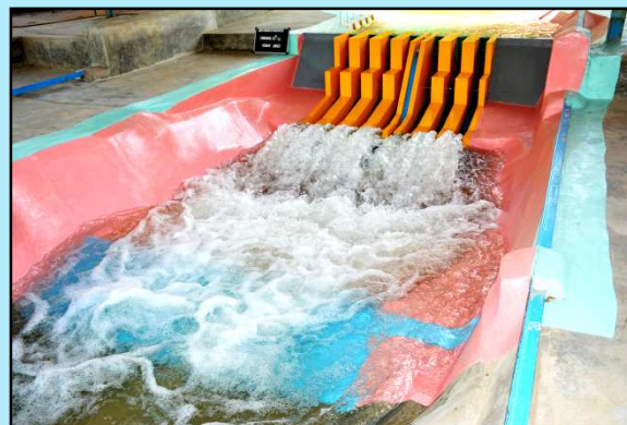
Punatsangchhu-II Dam Spillway, Bhutan
